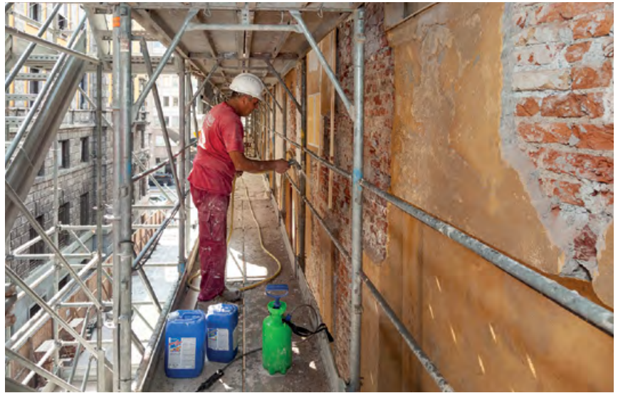
Before applying the render and skim coat, the masonry was consolidated by applying a coat of PRIMER 3296.
