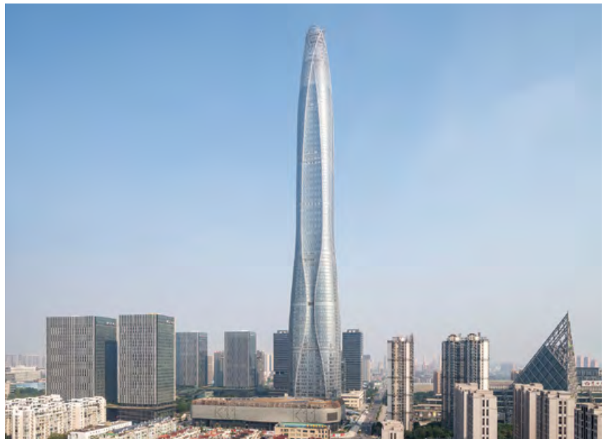
Tianjin CTF Finance Centre. Image: Seth Powers.
