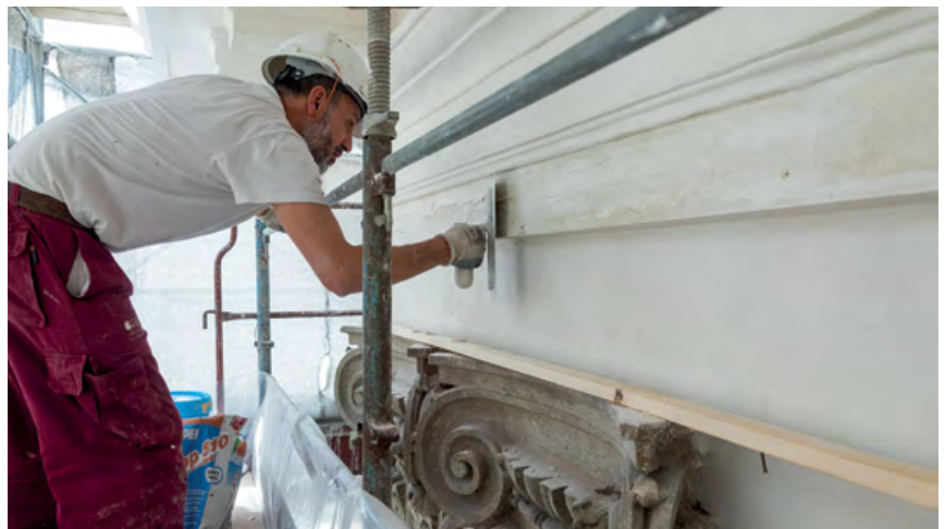
PLANITOP 510 fine-textured, lime-cement skimming mortar was applied on the external surfaces before painting them. When the render was made of lime, the product chosen was MAPE-ANTIQUE NHL ECO RASANTE CIVILE fine-grained, breathable, smoothing and levelling mortar.
