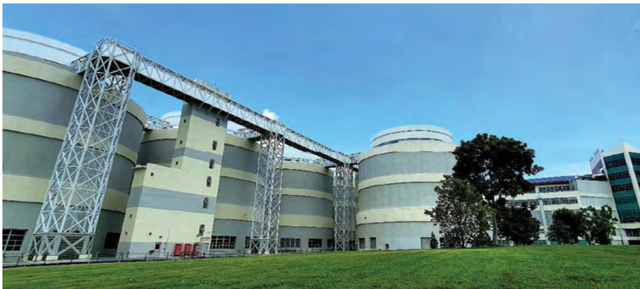
Process unit (digester) at Changi Water Reclamation Plant.
