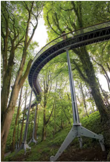
The Viper Elevated Walkway at the Newt in Somerset. Henry Fagan & Partners.
