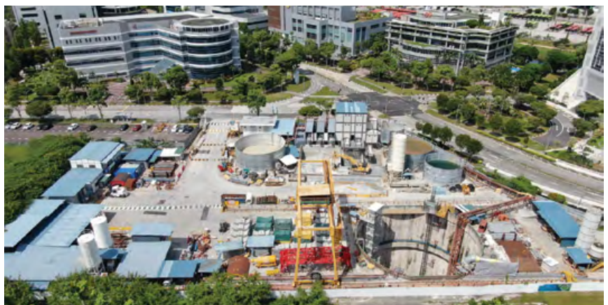
The Deep Tunnel Sewerage System (DTSS) Phase 2 Project will cover 100 km of the western part of the island. Image: CPG Consultants.
