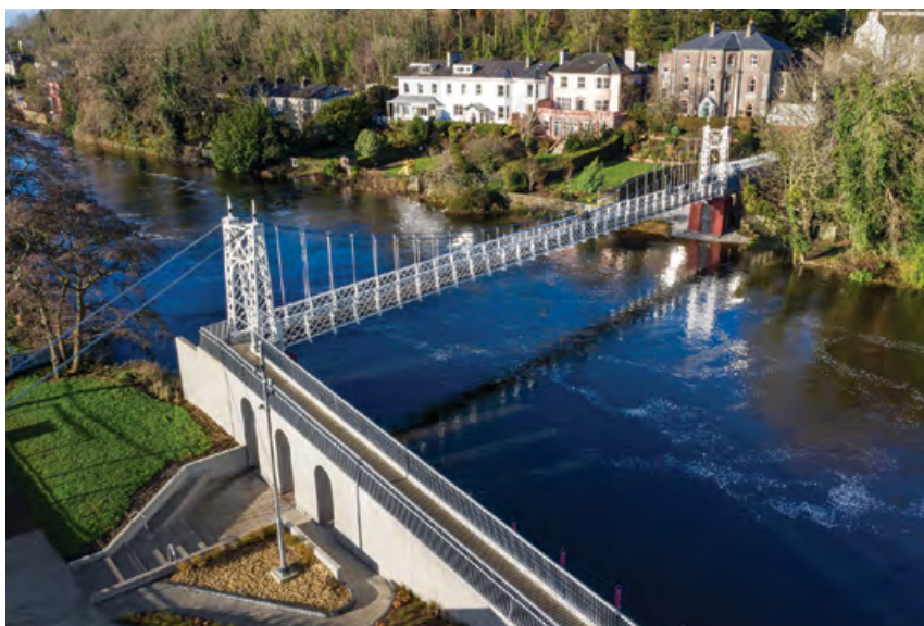
Repair and Rehabilitation of Daly's (Shakey) Bridge. Image: Michael Minehane.
