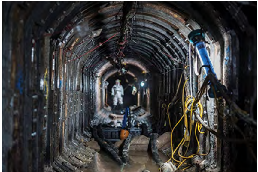
King's Scholars Pond Sewer Rehabilitation. Image: Roozbeh Shirandami.
