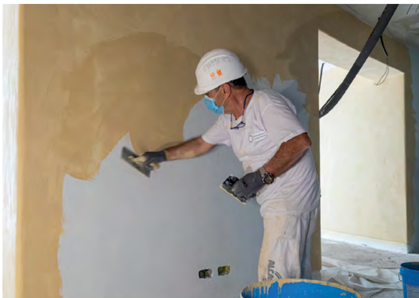
The walls in all the corridors, stair wells and stalls were finished off with SILEXCOLOR MARMORINO.
